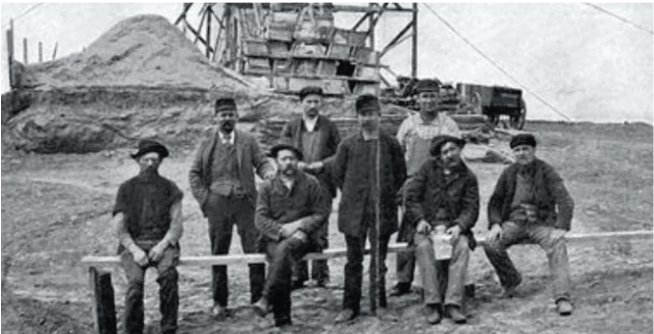
Gentlemen take a pause during construction
